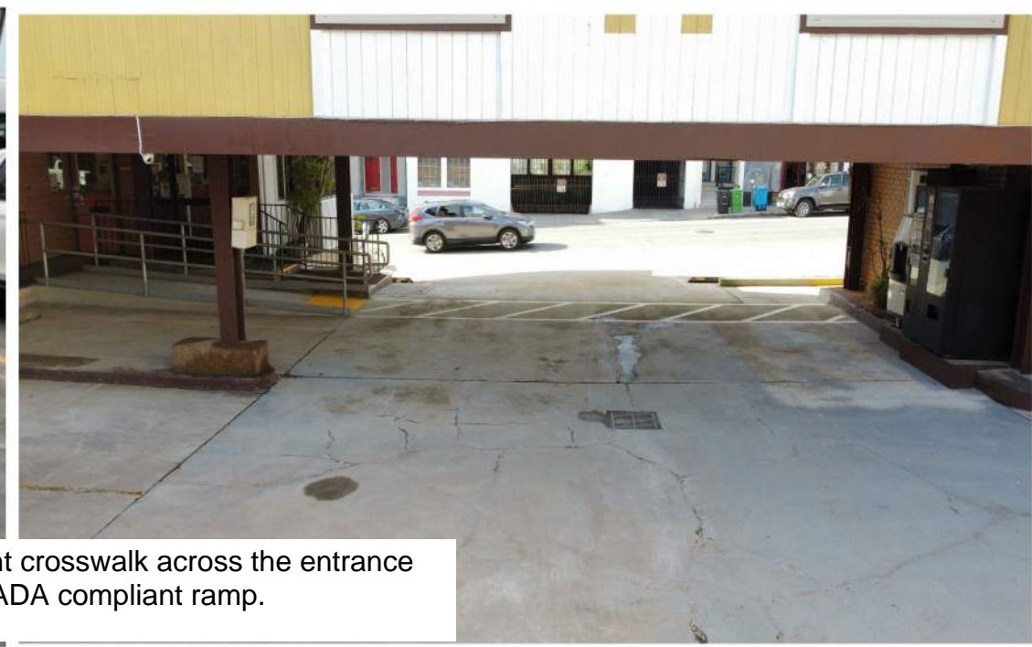
Pedestrian traffic had no designated access to the hotel office from the public sidewalk. Borrowing space from an adjacent parking stall, Protrk created a new ADA compliant concrete walk to navigate through the existing parking area.
