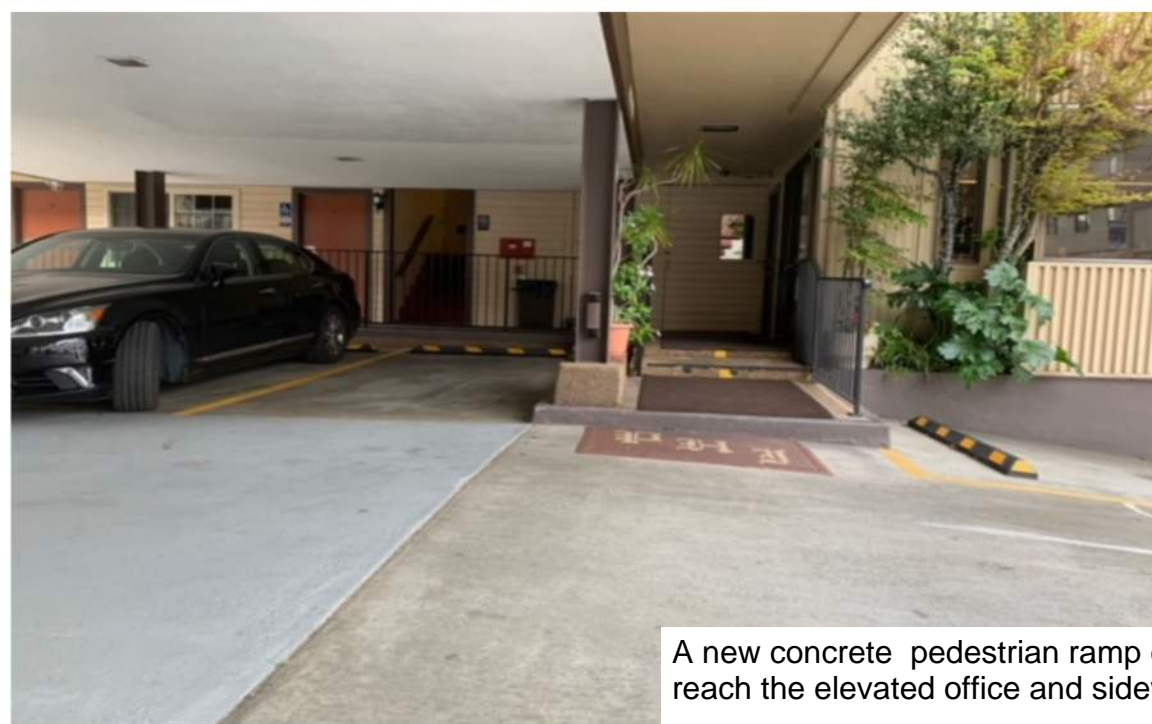
Protrk removed the existing non compliant walk across the front of the building and created a new ADA compliant walk.
