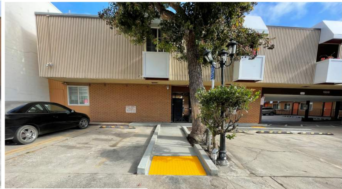
Pedestrian traffic had no designated access to the hotel office from the public sidewalk. Borrowing space from an adjacent parking stall, Protrk created a new ADA compliant concrete walk to navigate through the existing parking area.
