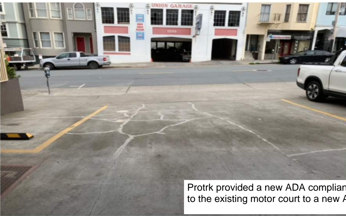
Pedestrian traffic had no designated access to the hotel office from the public sidewalk. Borrowing space from an adjacent parking stall, Protrk created a new ADA compliant concrete walk to navigate through the existing parking area.
